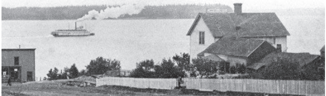
TOP: Interior and exterior restoration continues. BOTTOM: Haller House with the steam ship Farihaven in the background, circa 1890.
