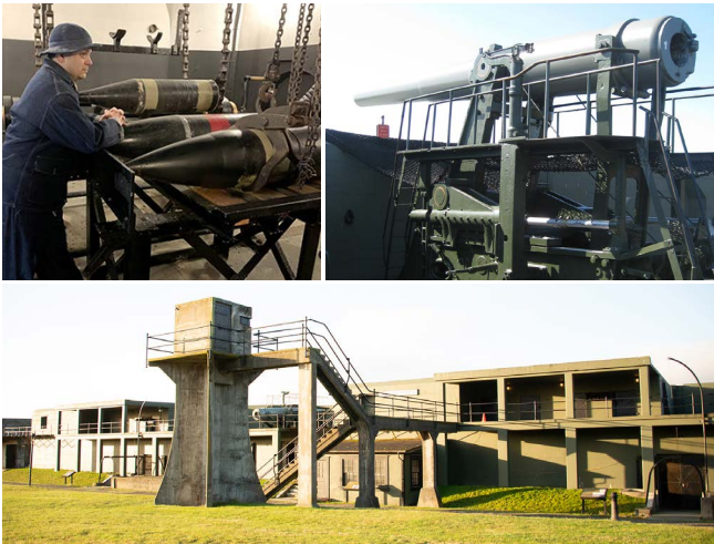
TOP LET: Worth Battery military reenactment. Photo: Sherrye Wyatt. TOP RIGHT: One of two 125-ton, 10-inch guns on retractable carriages. BOTTOM: Gun emplacements and raised fire control booth.
